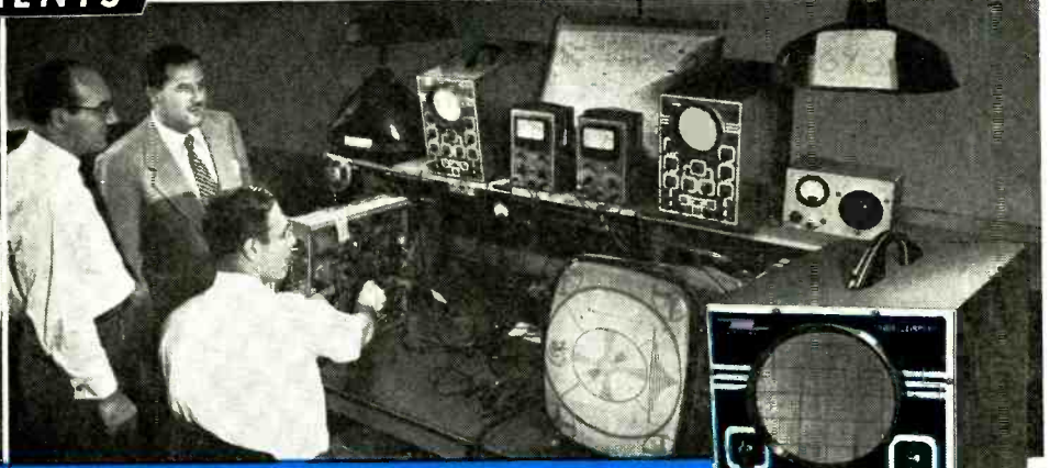
Frank J. Diehl, Majestic's Chief Engineer, and Harry R. Ashley, President of EICO, inspecting the use of the EICO Model 425 5" Push-Pull Oscilloscope, Model 221 Vacuum Tube Voltmeter and Model HVP-1 High Voltage Probe at the important Final Test Position on the Majestic Television production lines.
